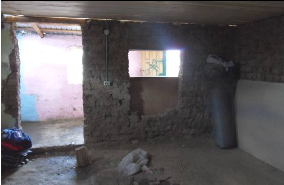
Fig. 13. Inside a house in construction from Oborul Nou.
