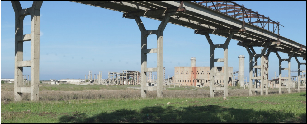
Fig. 2. Călărași –Siderca , the company that was supposed to be the largest steel factory of Europe at its time and for which a port was built, was never completed and now guards the exit road to Bucharest for about two kilometres. Demolition works took place in the last twenty years and are still ongoing.
