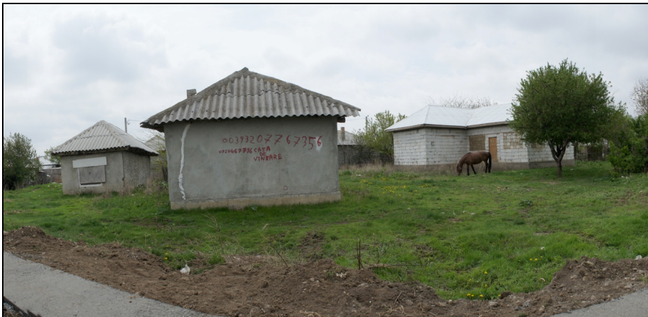
Fig. 16. House for sale in the Spoitor community from Călărași, the contact number written with paint on the wall is Italian.
