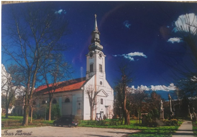
Photo of the Church, from the right side
