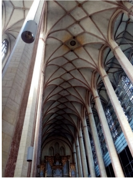
Fig. 1. Nave vault of St. Martin's in Landshut: an example of the rib pattern of 'Parleresque' vaults. (Photo: Jobbik Eszter)
