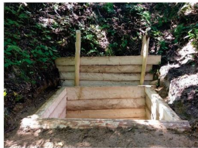
Fig. 8e. Modern cistern found on a nearby valley, personal photo.
