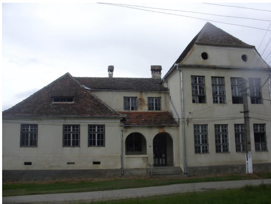
Figure 6 Western front of the school in Bruiu (Picture taken by the author, 2016)
