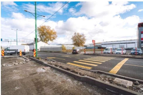
Fig. 10. Street improvement, decking and cladding (own source)
