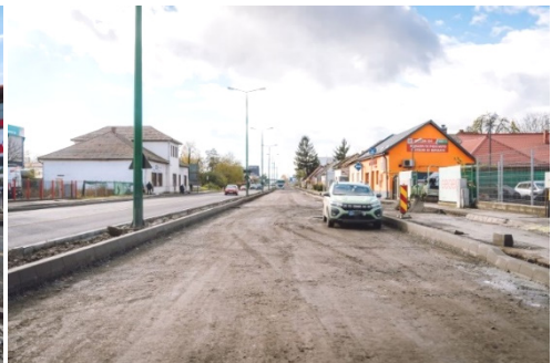
Fig. 11. Road network in work without asphalt pavement
