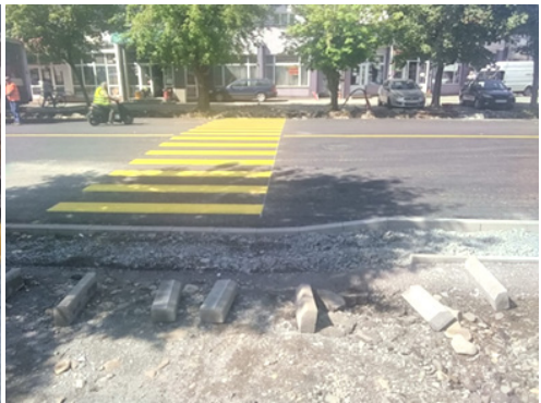
Fig. 5. Street improvement, decking and cladding (own source)
