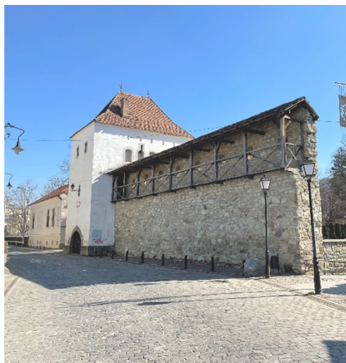
Fig. 3. The Coopers' Tower. Source: the author
