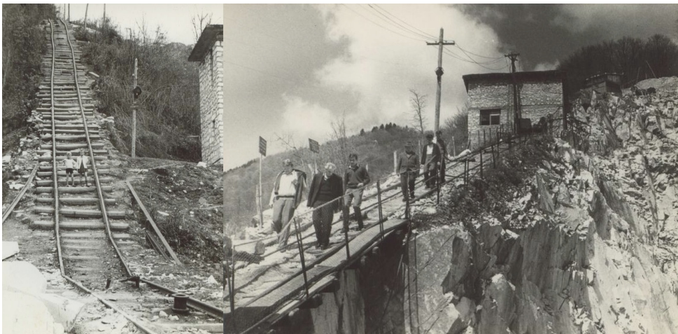
Fig. 12. The former inclined plane used for the lowering of marble blocks
