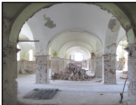
Fig.4. Inner image of D building
