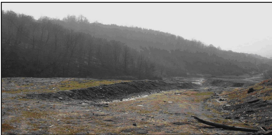
Fig. 3. Clough formed in the central part of the sterile dump. (Source: C. Nimară, 2011).
