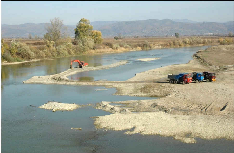
Fig. 13. Alluvial deposits extraction by artificial headlands
