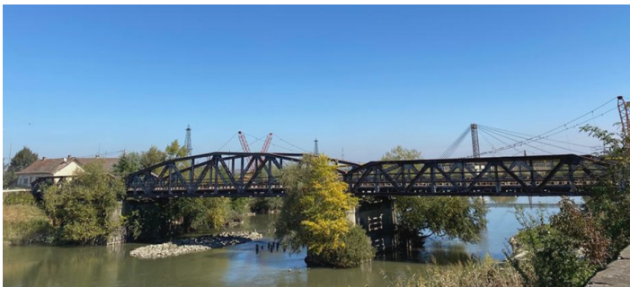
Fig. 4. The bridge over the Mureş River
