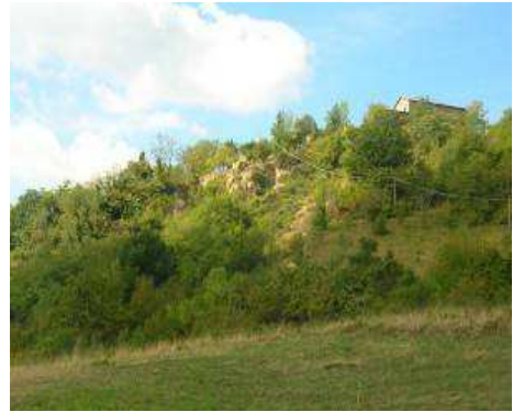
Fig. 8. Panoramic view of the upper part of the Ribecco landslide. Note the detached rock prisms near the landslide scarp, very close to the buildings of Ribecco.
