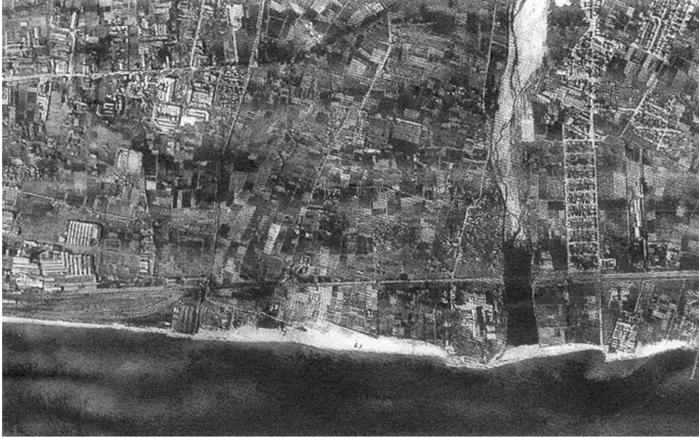
Fig. 2. The Besós estuary area before the rehabilitation.
