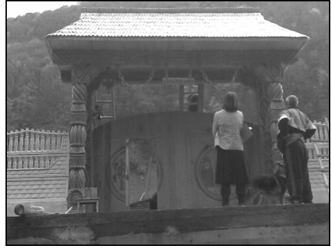
Fig. 17. Wooden gate built in Bihor County with rich decorations and a lot of new elements, combined with cement fence.
