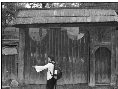
Fig. 14. Wooden gate from Budesti Village (Maramureș) with 3 pillars according with traditional architecture.
