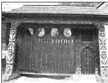
Fig. 15. Wooden gate from Sârbi Village (Maramureș) with 5 pillars according with traditional architecture.
