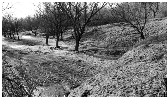
Fig. 3. Toe of a more recently reactivated landslide body on the DC 79 landslide.
