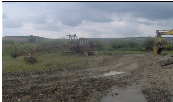
Fig. 6. Correction works on Valea Mărului (September 2008)
