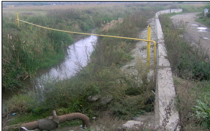
Fig. 2. Support wall on Lujerdiu River, in Fundătura village (September 2008).
