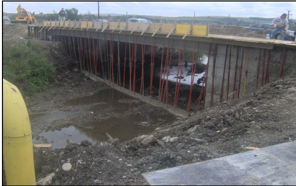
Fig. 3. Rebuilding of the road bridge on Lujerdiu River (Fundătura, September 2008).
