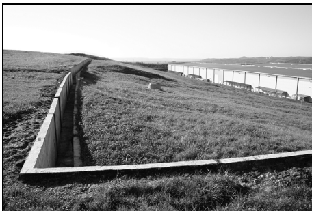
Fig. 15. Countermeasures above the factory building, Dumbrăvița (2012).
