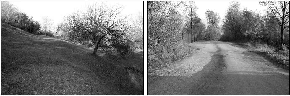
Fig. 6. Rotational landslide toe (left) illustrated in fig. 7, and damage to the road crossing landslide area on the southern Unguraș slope (right) (2012).
