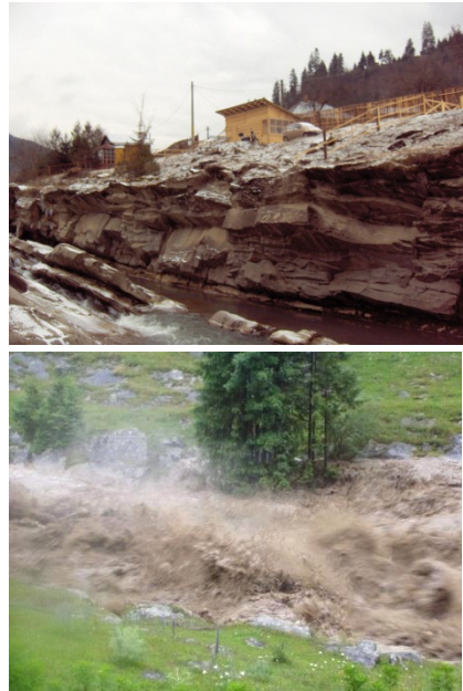
Fig. 2. The left bank of Tarcău River 25 m upstream of Cazaci gauging station (up); the water level during the historical flood in the same location (down—photo: Iulian Găină).
