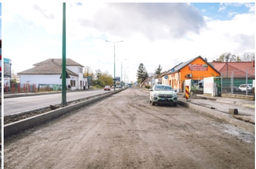
Fig. 11. Road network in work without asphalt pavement
