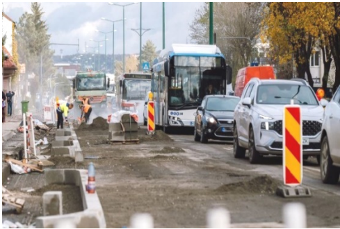
Fig. 8. Road resurfacing works ( own source)
