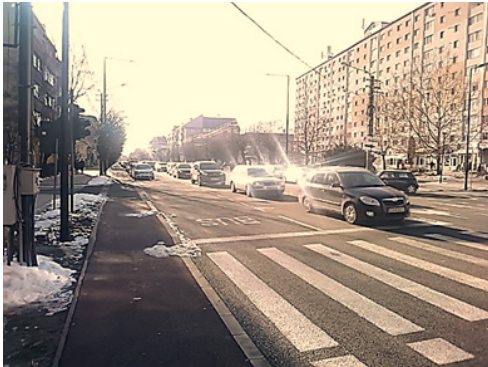
Fig. 12. Final layout of the street works, bike path
