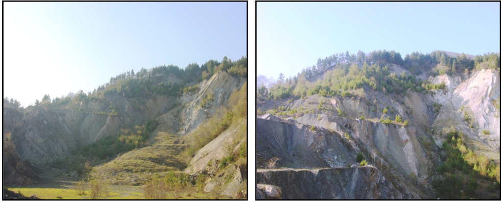
Fig. 5. Victoria coal pit and the landslides on its slopes. (Source: Nimară, 2011).
