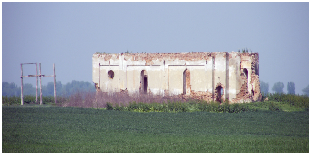
Fig. 20. The ruins of the Orthodox Church in Filiu village, Brăila County, destroyed by floods in 1970 (Source: https://commons.wikimedia.org/wiki/File:2013_-_Biserica_din_satul_Filiu_comuna_Bordei_Verde_in_ruina_-_Exterior.png )
