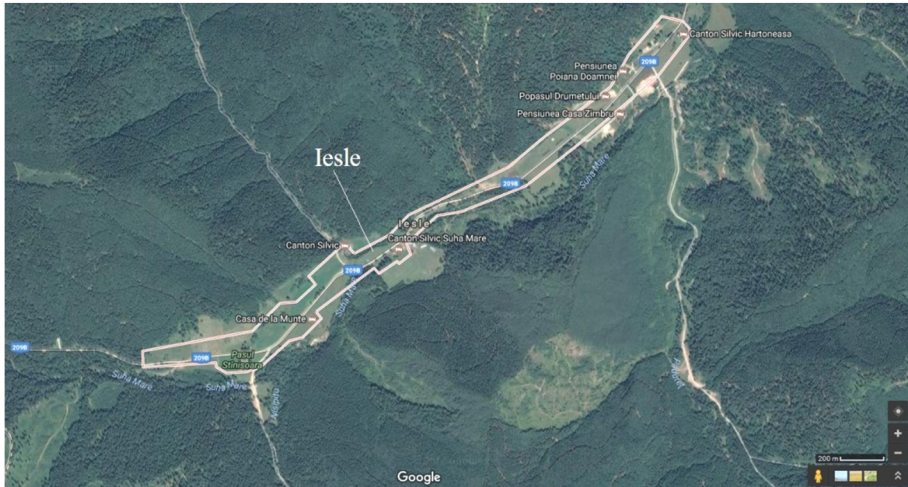
Fig. 15. Settlement with whole built-up area with seasonal living. The case of Iesle village, Mălini commune, Suceava County, Romania ( Source: Google maps )
