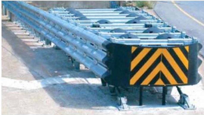
Figure 11. Trapezoidal road safety crash cushion [12]
