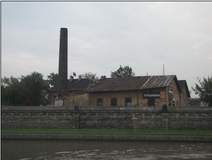
Fig. 9: The old power plant of the Podgórze District in Krakow, view from the Vistula River (photo: Andreea Iacob, July, 2011)
