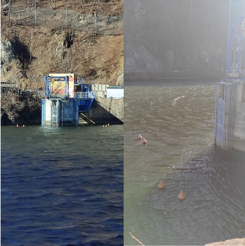
Fig. 2. Tarnița raw water intake and its protective buoys
