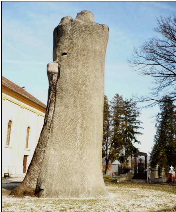
Figure 3. The image shows the remains of the dead oak, with the trunk encased in the concrete sarcophagus. The remaining original bark is visible on the left side of the photo.
